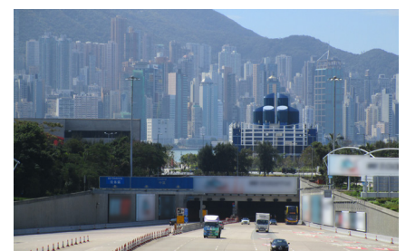
図5 Western Harbour Crossing (WHC)
